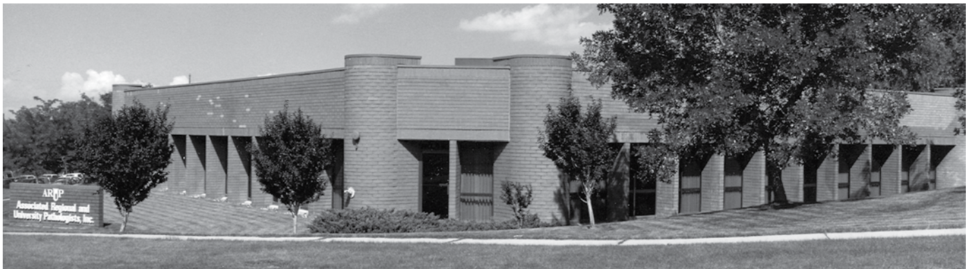
ARUP's first building at 390 Wakara Way in Research Park; ARUP OUTGREW ITS FIRST HOME WITHIN THREE YEARS.
